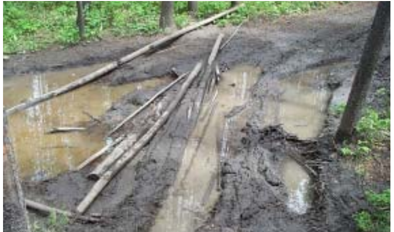
ATV Damage on the Pioneer Lakes trail, Gallatin National Forest (Courtesy Phil Knight)
